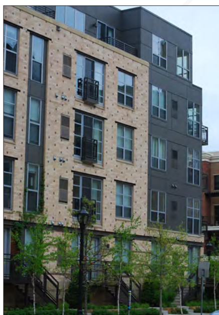
Fenestration pattern in light colored brickwork framed by dark panelling organized around vertical proportion.
