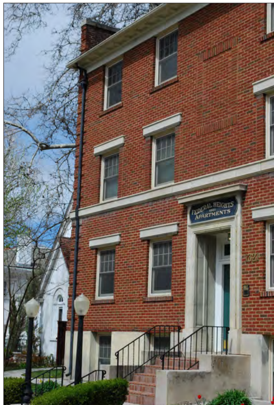
Federal Heights Apartments
