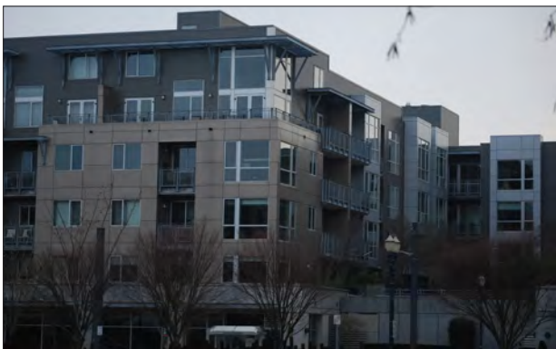
Designing for a variety of complimentary street facade elements can integrate private terrace space and achieve a distinct sense of human scale.
