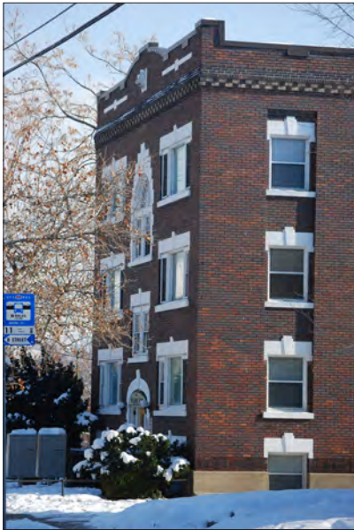
Wilshire Arms Apartments
