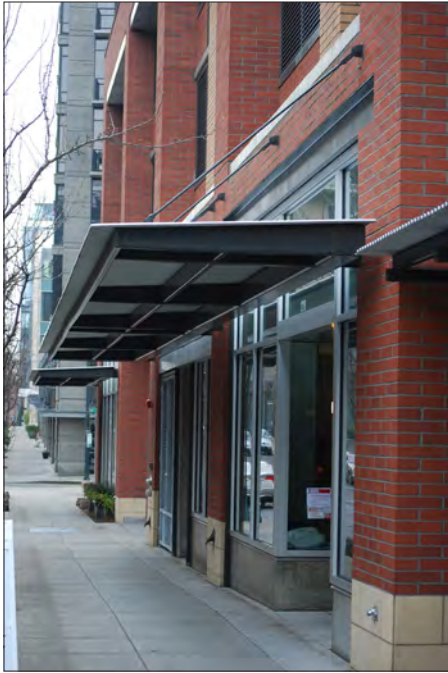
Durable materials frames and support shade provided by deep window reveals and fixed canopies for street level retail and sidewalk.
