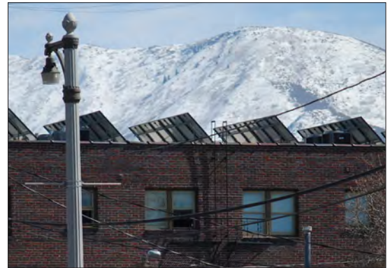
Building utility locations can have unanticipated consequences.
