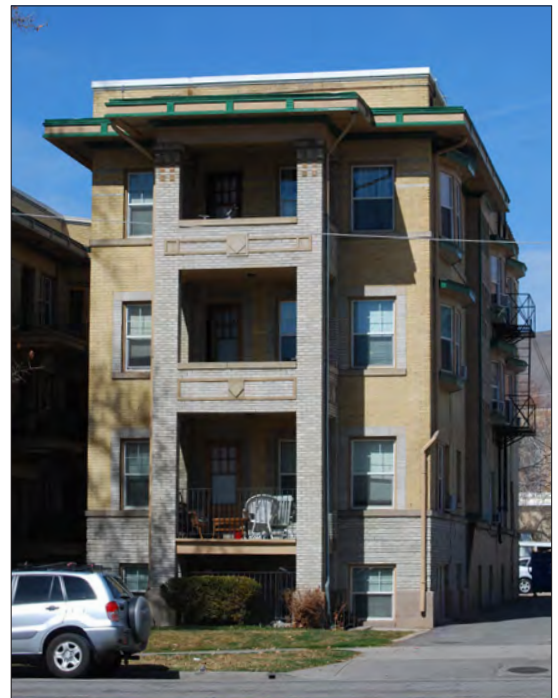
A principal projecting wing of the street facade, combined with projecting balconies, can effectively maintain a distinct human scale in a much larger building.
