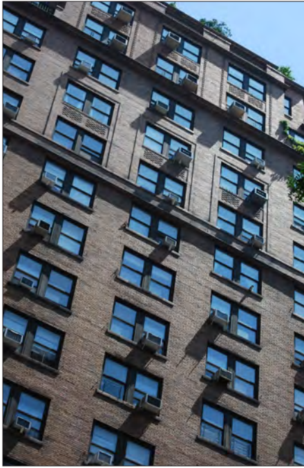
Retrofitting equipment individually can have a significant visual impact on an older building.
