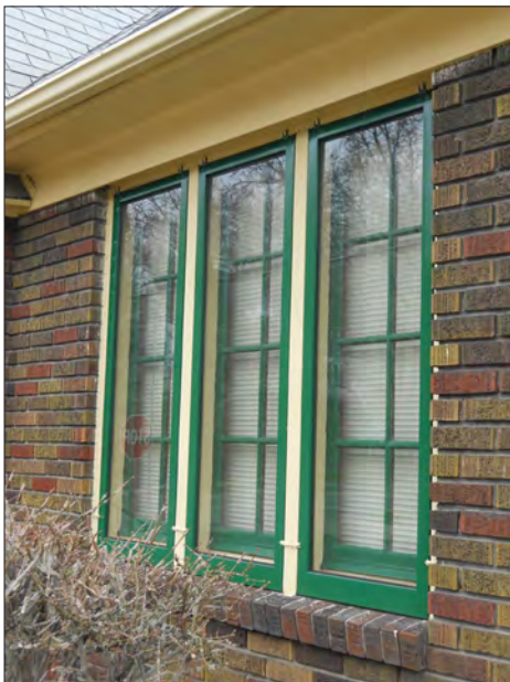
Historic wood windows, enhanced with a traditional design of external storm window, will generally outlast and outperform a replacement window.
