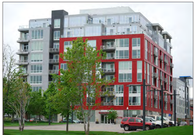
Balconies, modeling, varied fenestration, stepped back upper floors and color, employed in composition to reduce the apparent scale.
