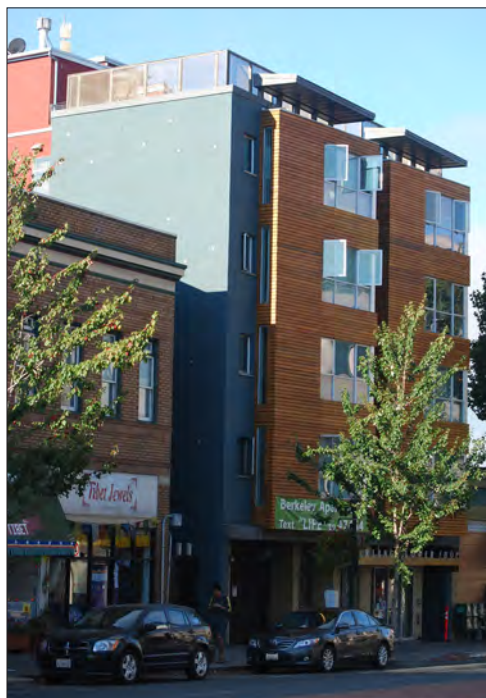
Recessed garage access from the street with minimal interruption of the street frontage.
