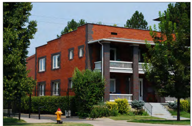
The traditional characteristics of the thermal mass of solid materials, natural ventilation and the south-facing shade provided by a shared arrangement of balconies combine to moderate the extremes of climate without mechanical means.
