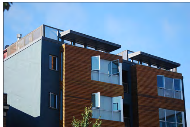
Recent apartment design creatively using traditional materials, open spaces and natural ventilation.
