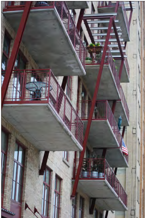
Window proportion and detailing are accentuated by rising, projecting balcony tiers, and their decorative structural ironwork.
