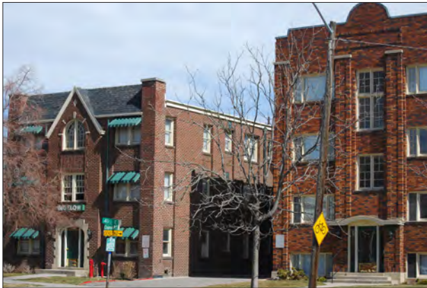
Despite contrasts in height and architectural style, the solid to void ratio and window scale and proportions help to establish an affinity here.
