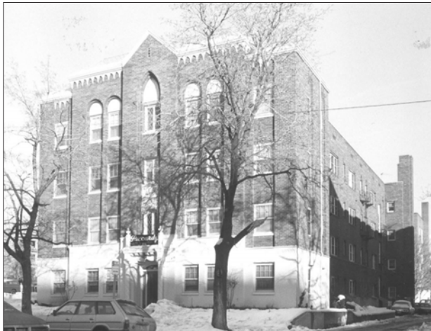
Picardy Apartments, c. 1928, Salt Lake City, Salt Lake County. This central-entry apartment building is highlighted by a terra-cotta base and a cornice of blind arcading.
