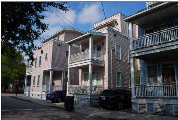
Limiting street facade sheer height, combined with projecting balconies, help to reinforce a sense of human scale.
