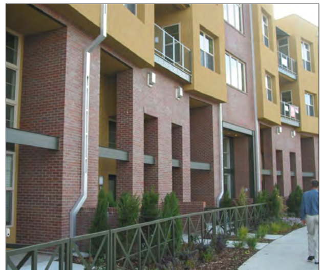
Deeply recessed windows and doors on lower floors create a strong sculptural base for the articulation of the facade above.
