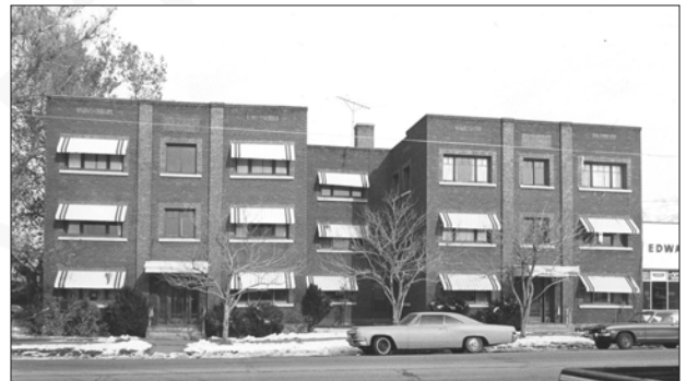
Rose Apartments, 1923-24, Ogden, Weber County. This is a brick masonry “C”-shaped apartment building containing entries in the wings.
