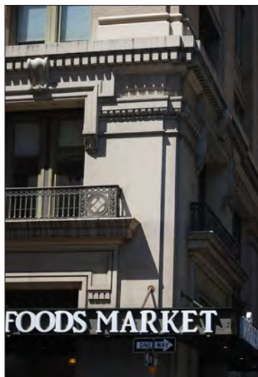
Signs and lettering design can reflect and also enhance the building.
