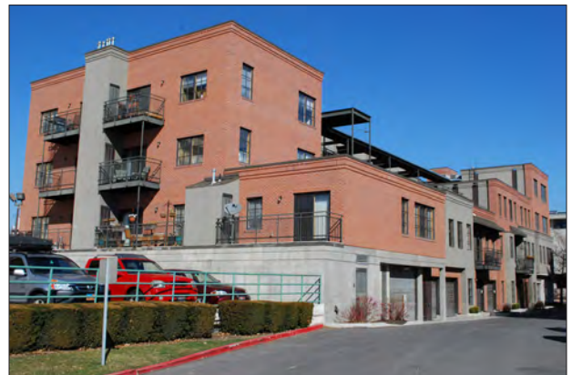
Recent multifamily design composed with varied volumes and massing, private and social open spaces and constructed using solid durable materials.
