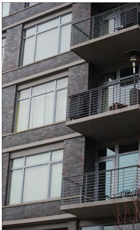
The design of a projecting balcony arrangement should still provide the opportunity for architectural creativity and detail.
