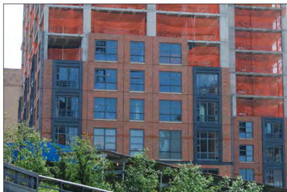
Contrasting dark vertical window bays frame a subtly vertical fenestration pattern in this brick facade.
