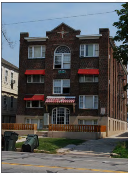
Central approach, entrance and axial 'pedimented' bay help to enhance the coherent, symmetrical contribution to the street.
