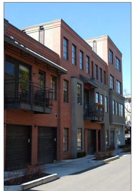
Stepping down the height of the street facade introduces a more intimate scale and terraced private space to the rear.
