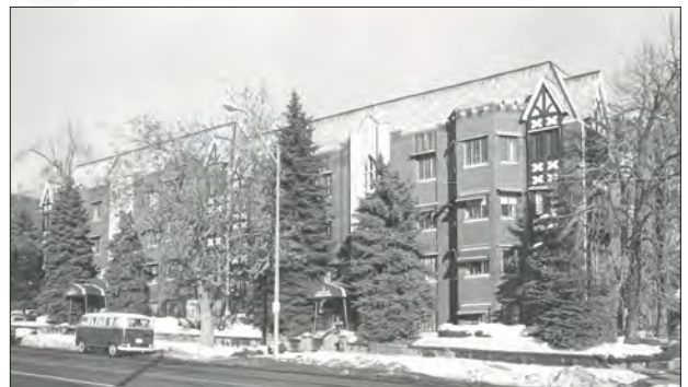
Chateau Normandy Apartments, c. 1929, Salt Lake City, Salt Lake County. This stepped, horizontal block of apartments illustrated the period revival style with its crenellated bays and half-timbering.
